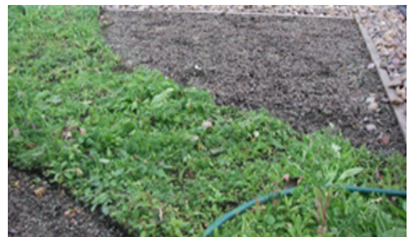
Green Estate substrate installed on wildflower roof.
